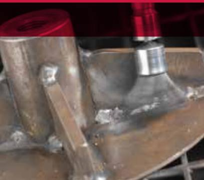
Cleaning hard-to-reach fillet welds on a gusseted base plate.
