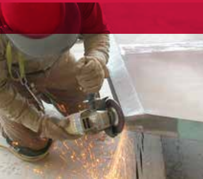
Grinding on a platform for weld preparation.
