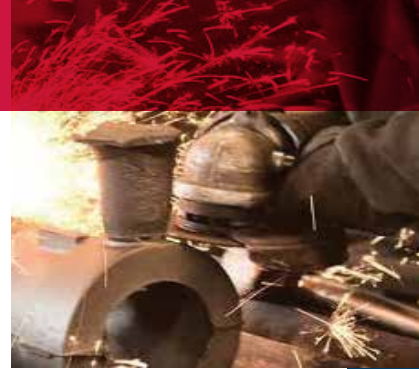
Riser removal with a type 27 grinding wheel.
