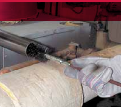
Cleaning boiler pipes with a flue brush.
