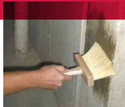
Applying waterproofing material with a masonry brush.
