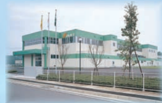
Mie Plant (TA & IT Plant)
