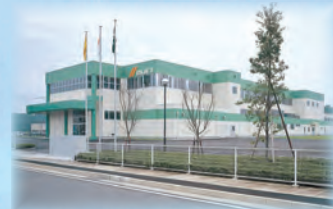
Mie Plant (TA & IT Plant)
